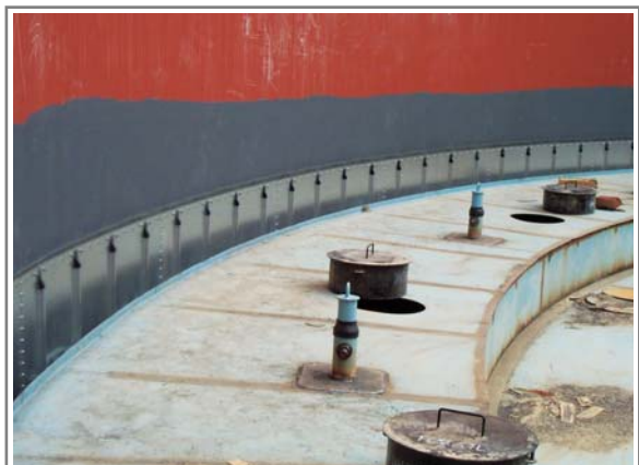
Shoe Plate after Installation
