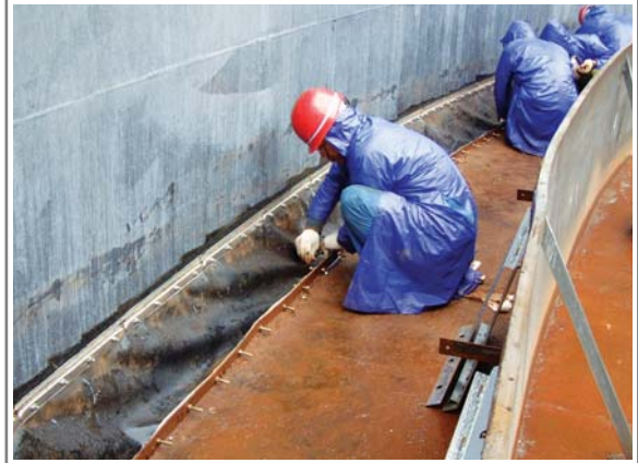
The installation of continuous seal (Tank Dia 60M-China oil company)
