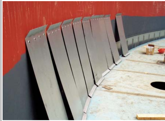
The Wax Scraper seal is ready to be installed at China oil company between tank shell and pontoon
